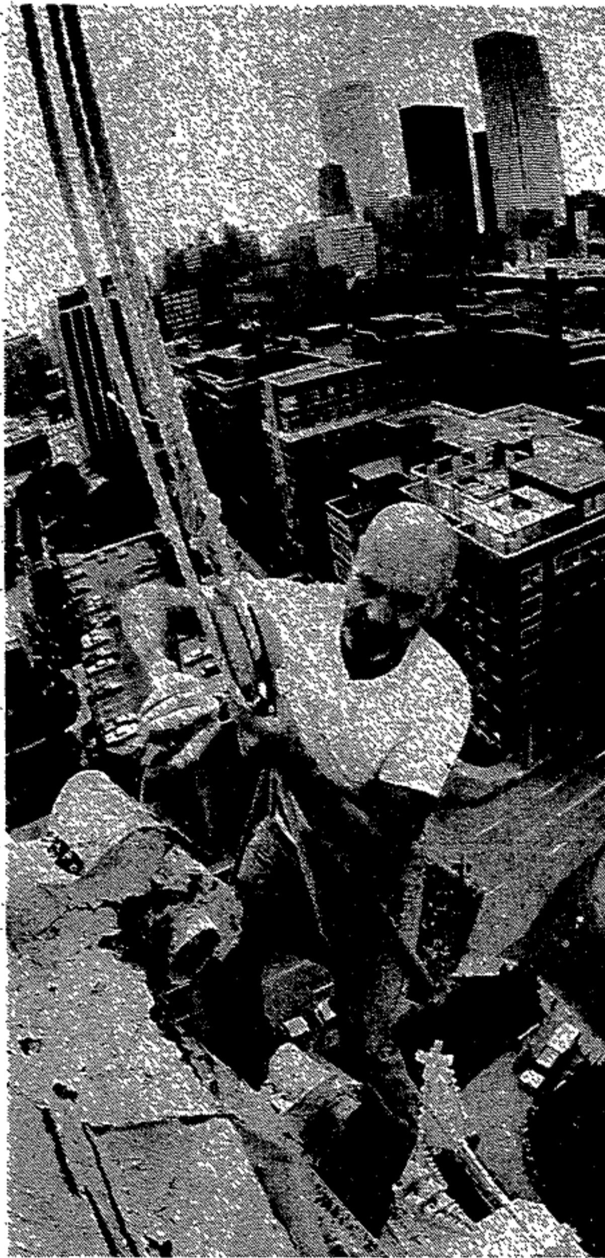
A BOSUN'S CHAIR — just enough to seat him — is all that supports Bill O'Connell as he works on St. Michael's spire. Wooden ladder was built to top of spire and a block-and-tackle attached to the cross supports the workers' chairs.
